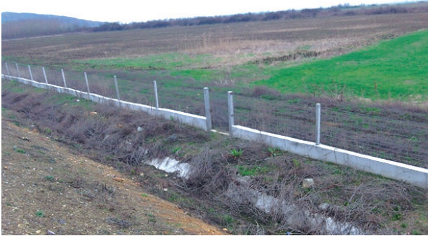
Fig. 1. Concrete walls for protection of vehicular turtle mortality at Trakiya Motorway. Note the gap in the wall where the service door is mounted
